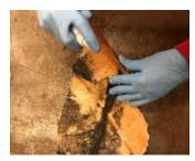
5. Spray accelerator (part 2) to cloth & adhesive area.(Hold for 1 minute to cure)
