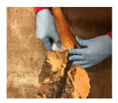
4. Apply adhesive (part 1) to entire crack & cleaned surfaced area.
