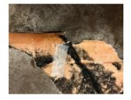
2. Cut the enclosed fiberglass cloth 1" wider than the crack. adhesive area must be dry
