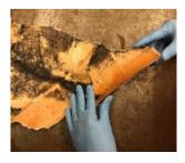
3. Align the crack & place Fiberglass cloth over it w/ at least  $\frac{1}{2}$  on both sides.
