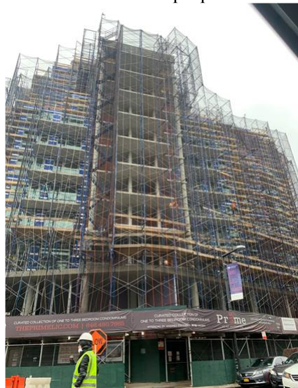
View of typical scaffolding used for the erection of exterior wall systems that will be eliminated with the introduction of Portal Wall Technologies
