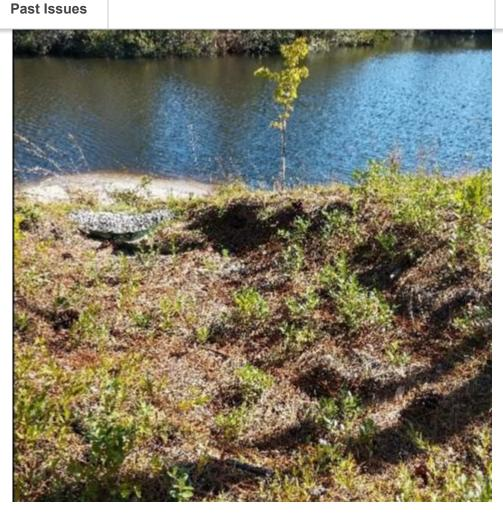
A sinkhole is formed when high volumes of water wash away subsurface soils creating voids and weakness above. Erosion can also occur from simple wave action undermining the lower part of the pond bank over time.
