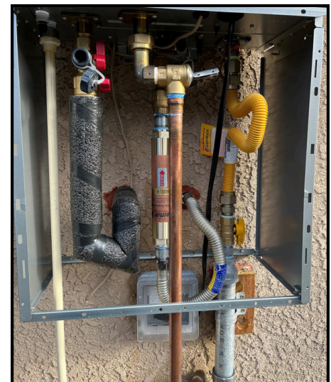
Superior unit installed on a tankless water heater
