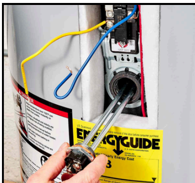
New, Scale Free Heating Element
