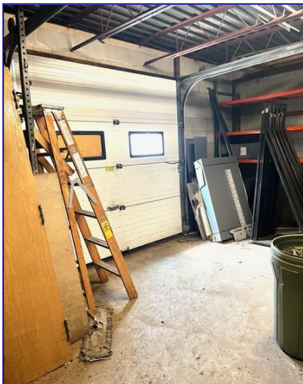
Overhead Loading Door
