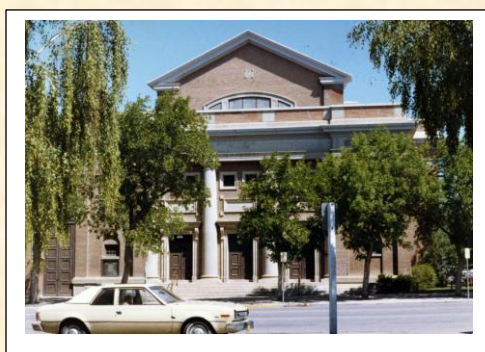
4 th Avenue façade before Senator Buchanan Chapel was built
