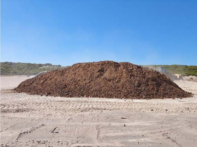
Stabilised drilling mud and cuttings stockpile.
