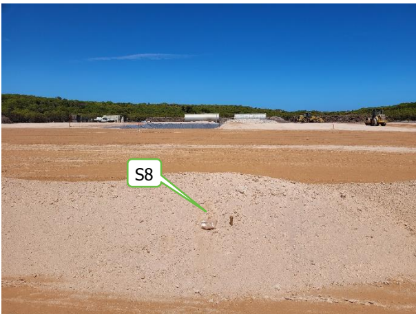
Imported material and S8 location, 15 March 2022.
