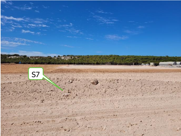
Imported material and S7 location, 15 March 2022.
