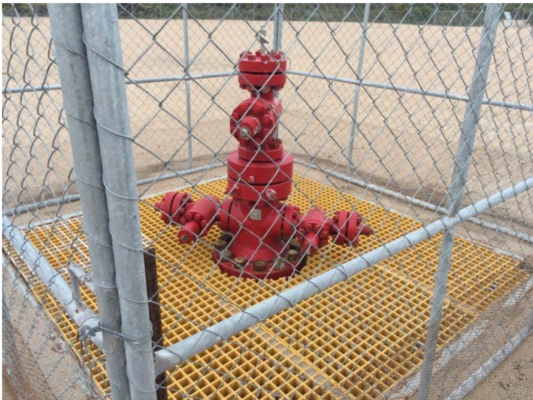
Figure 3: Example Wellhead Cellar Covered and Fenced
