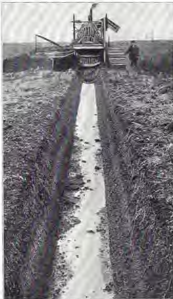
DITCHING MACHINE DIGGING LATERAL DITCH AT DELTA FARMS.
