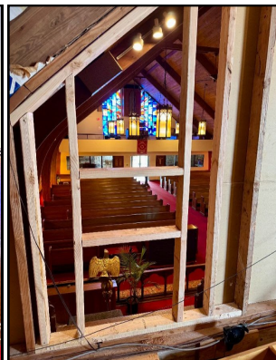
Photos show the old speaker panels being removed and framed for air ducts.
