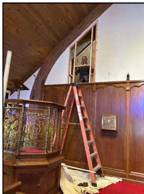
Photos show the old speaker panels being removed and framed for air ducts.
