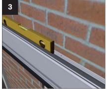
Lift the box gutter back into position, check levels, and then mark the wall (through the pre-drilled holes) ready to drill the host wall and grind out for the flashing.
