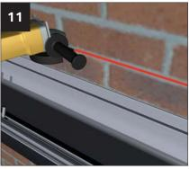
Mark out and grind a channel in the masonry for the flashing - blow out any dust in the
