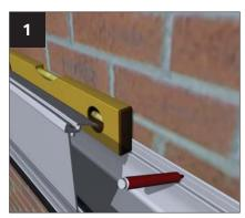
Offer the raised back or special box Lift the box gutter down to the ground and gutter into position. Carefully mark onto turn it around. Drill through the aluminium the aluminium leg against the host wall leg (that abuts the host wall) at the prethe position of each fixing - use 600mm marked positions. Whilst the box gutter maximum centres.
