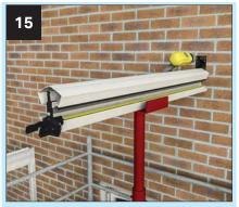
Prop ridge in position using suitable Using the roof rise height supplied set the supports, centralising between eaves ridge and fix the bracket to the host wall using the appropriate fixings.
