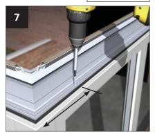
using for example, 38mm x 4.8mm screws in the position shown. Fix down at 450 centres and within 200mm of each corner. For 60mm frames use the inner eaves extrusion line and outer line for 70mm frames. Always screw down. (Not supplied)
