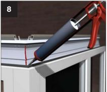
Securely fit the eaves beam to the frames Once the eaves beam is secure, run a bead Whilst ensuring that its level, drill through of silicone down the joint where the eaves beam sections meet and where the eaves abuts the host wall.
