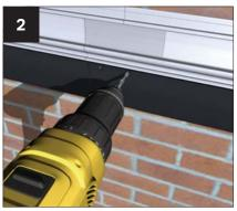
Drill through the top edge of the aluminium box gutter at 600mm centres .A fixing must be positioned within 50mm each side of the joint.
