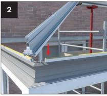
If not already attached, attach the glazing bar end cap fixing blocks - as access restrictions may prevent easy fixing later. NOTE: These 'snap out' of the end caps when dispatched from the factory. remove nuts on eaves beam. Fit hip bars onto bolt sat eaves end and hand tighten nuts.
