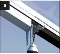
Take the transom bracket (CHA001) and attach using two 4.2 X19mm self-drill pan head screws (supplied). The back edge of the bracket should butt up to the under cladding.
