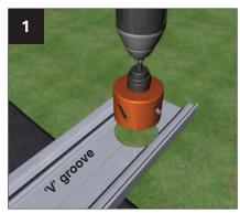
Decide the position of the gutter outlet by lining the extrusion 'v' groove up with the centre of the hole for the down pipe. Using a 73mm dia hole saw, cut the hole for the down pipe in the lower section.
