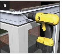
Using the pre-drilled pilot holes, drill two Securely fit the two M5 x 12mm taptite 4.5mm holes through the corner cleats.
