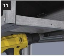
Attach L-Shaped frame using one of the Check the frame is level and and fix either three positions on the bracket, use 4 x13 on or below fascia wing using 4.8 x 32 selfdrill screws provided.
