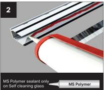
Seal underside of top face of glazing end profile as shown (PVCu version of end profile is shown - if aluminium glazing bar top caps, this end profile is also aluminium).
