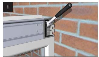
Where the eaves beam sits against the host masonry wall, it has a structural moulding attached to the eaves beam. This has three fixing positions cast into it to allow attachment into masonry choose the hole that directly lines up with solid masonry and drill a 10mm hole into the host wall. Attach the structural moulding the moulding attaches to the eaves beam.
