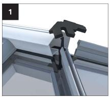
ENSURE THE GLASS IS CLEAN AND DRY BEFORE FITTING. Peel back protective film from weathering shield and position (adhesive face down) on glass, locating around the ridge and the hip bars. Press down firmly.
