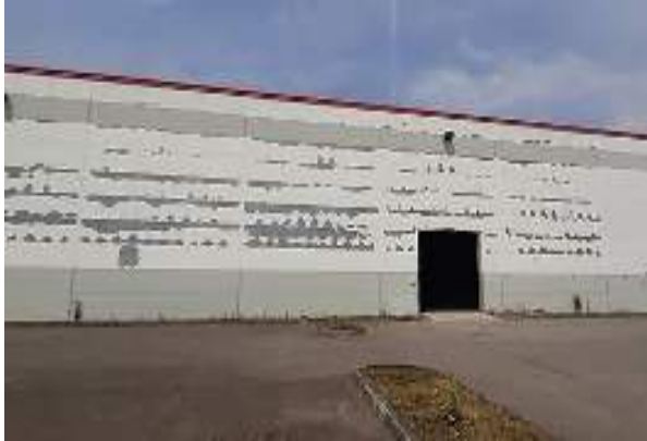
Photo 1: Unit 1A external.
