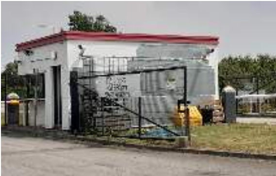
Photo 13: Security cabin (east).
