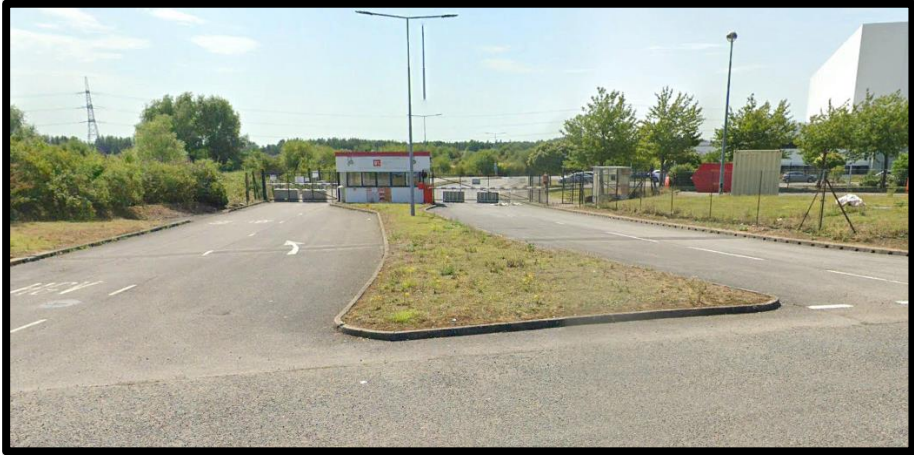
Main vehicle security entrance
