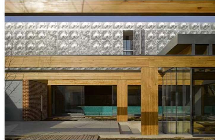
Ladderstile House, London
