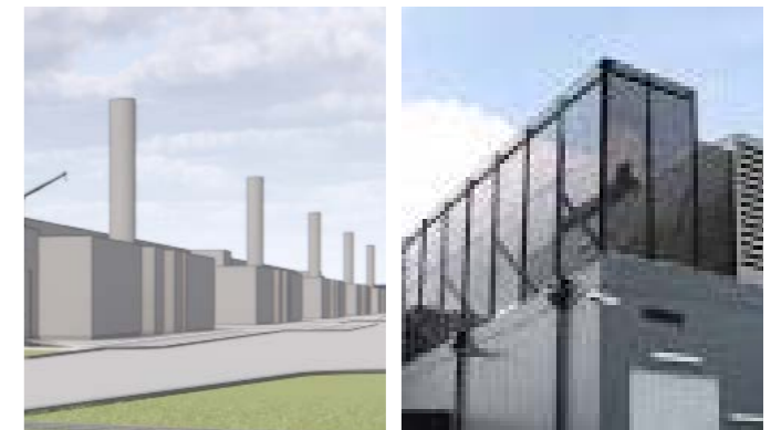
GENERATORS AND OTHER EQUIPMENT
