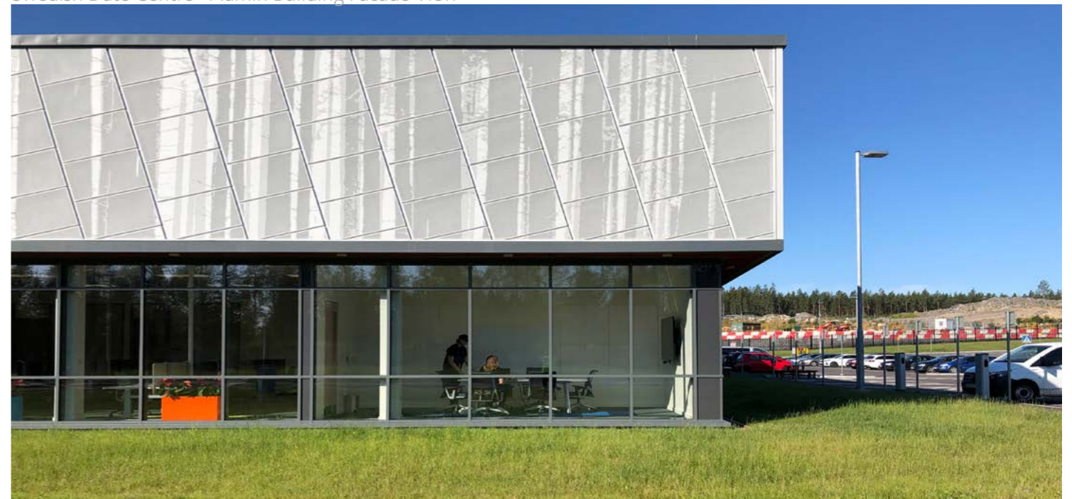
Swedish Date Centre - Admin Building Facade View
