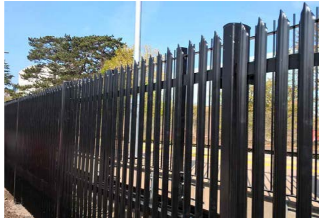
Perimeter security fence finished in Jet black, RAL 9005
