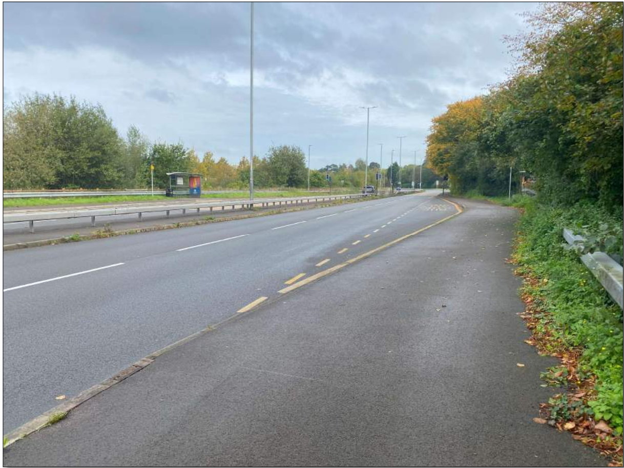
Figure 5.9 Bus Stop on A48
