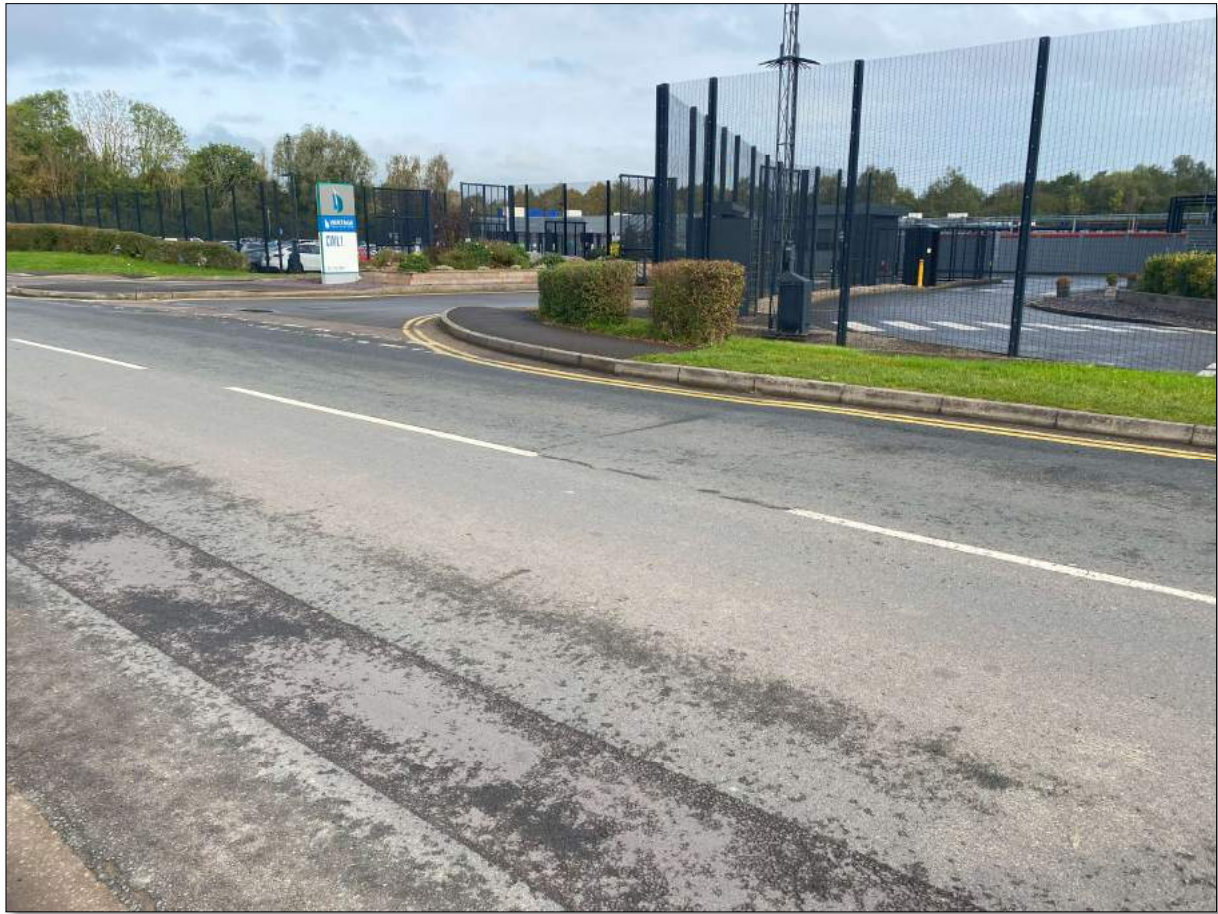
Figure 5.6 Access to Vantage DC
