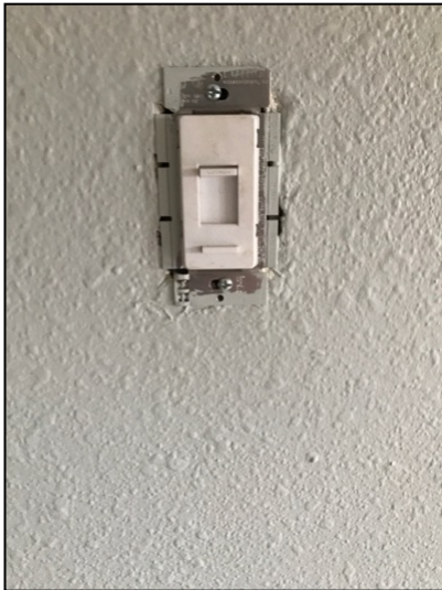
Switch cover plates missing on hallway light.
