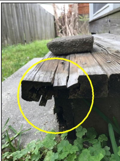
Rotted wood on steps East side of patio.
