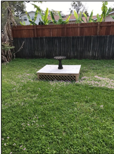
Possible drainage/clean out issues with “structure” built over drain.
