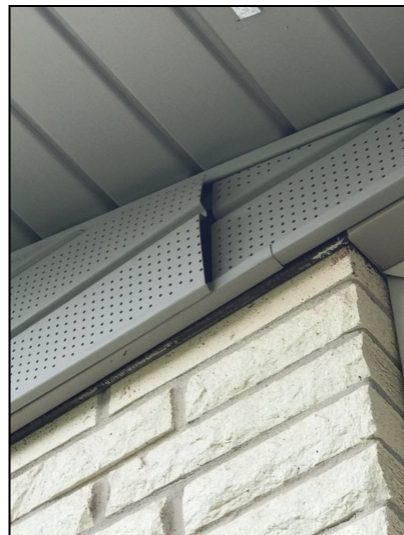
Some siding needs to be reset at front gable.
