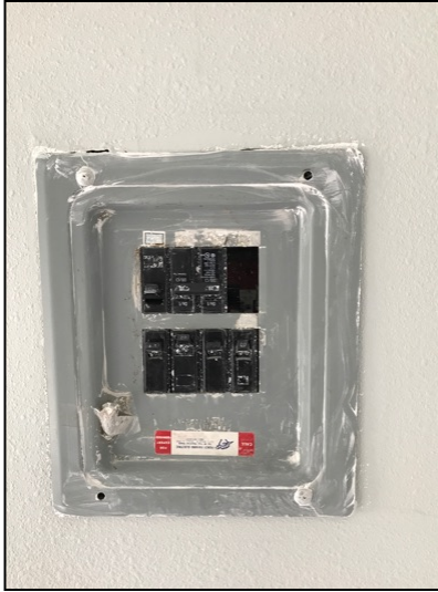
Sub panel door missing on sub panel behind garage.
