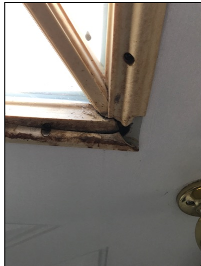
Window casing in door leading to open patio damaged.
