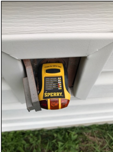
Outlet at rear of house not working. Outlet on non-enclosed patio section not GFCI protected.
