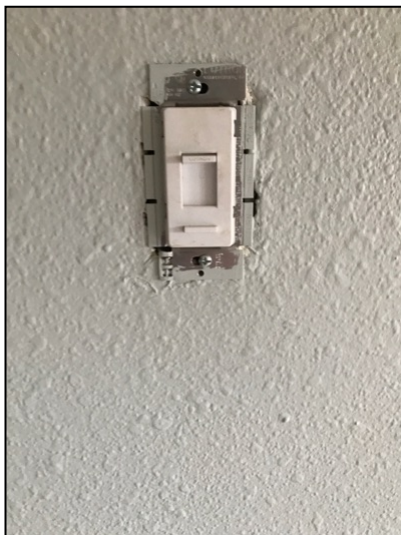
Switch cover plates missing on hallway light.
