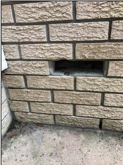
Brick missing by front door.
