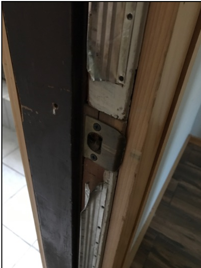
Door jam damaged leading from living room to fireplace room.
