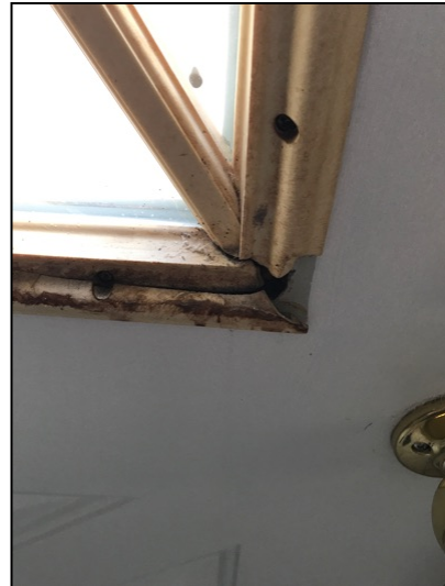
Window casing in door leading to open patio damaged.
