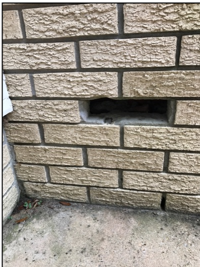
Brick missing by front door.
