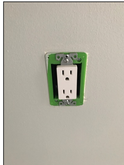
Missing outlet covers in room behind garage and room with fireplace.
