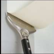
scraping off wall paper
