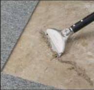
smoothing the floor surface
