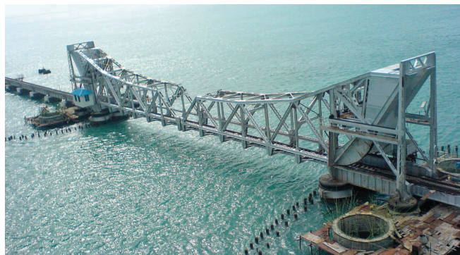
Infrastructure Investments Will Fuel Growth in Middle-to-Low-Income Countries. Annai Indira Gandhi Road Bridge – Gulf of Bengal, India.
