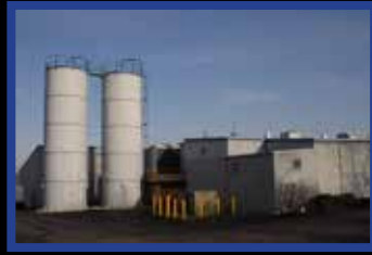
Plastic molding pellet silos provide ample raw material to meet any change in demand of molded product
