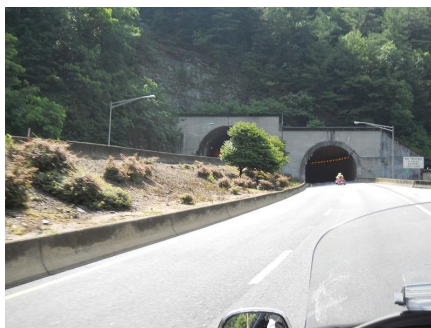
Tunnel thru the mountain
