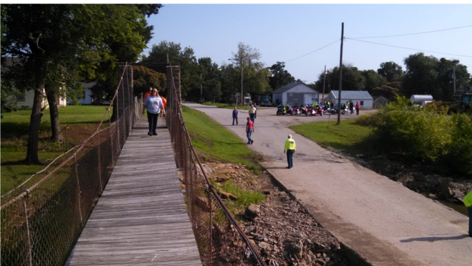
Oldest suspension bridge in Kansas
