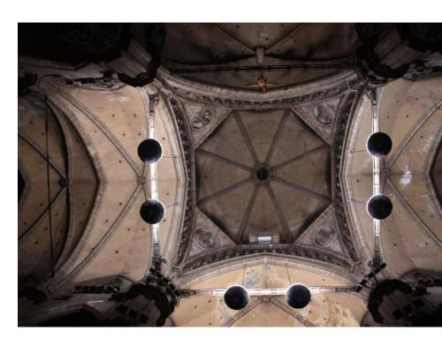
The light is directed upward, specific to working on ceiling, only illuminates the work area.
