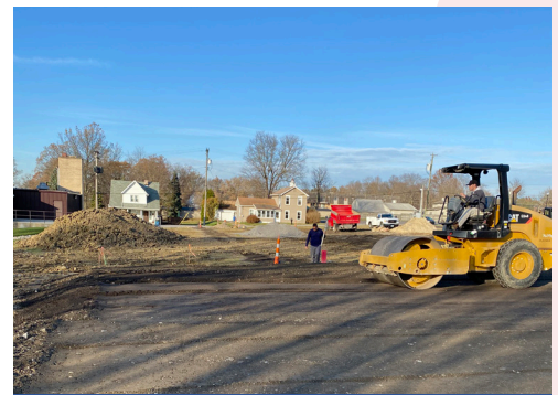
Construction is underway for the new Multi-Jurisdictional Opioid Education and Workforce Development Center at Gazebo Park.
