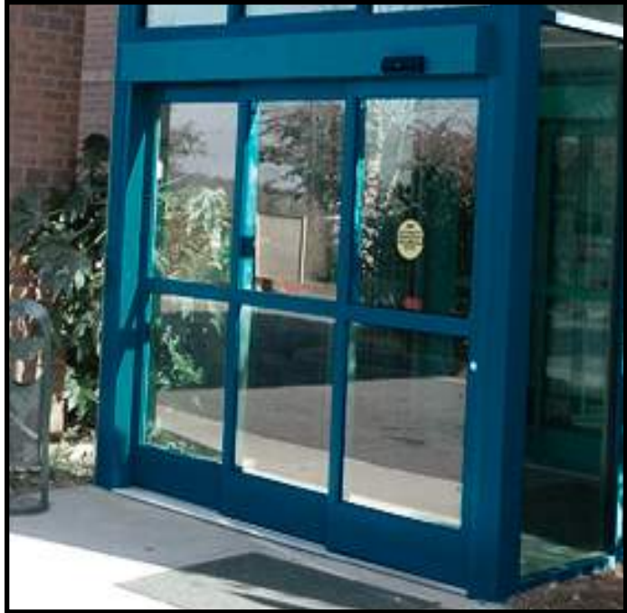
AUTOMATIC SLIDING DOOR TORMAX: TX9430 Full breakout telescoping slider RH, SX-SX-SO Conf: color: PMS 2188
