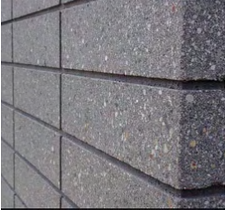
BASE BUILDING AND LOW WALLS: MASONRY Surface Matters masonry: color: Fire Ash, dry block. Stack bond.
