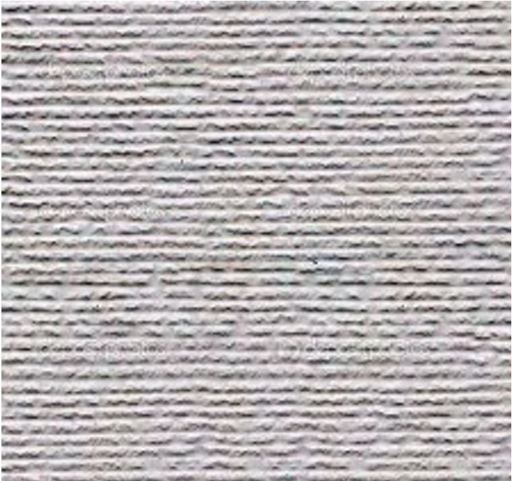
BASE BUILDING: GROOVED STUCCO Horizontal and vertical parallel grooved stucco, w/ 4'-0" O.C. black expansion joints. Color: Benjamin Moore (low VOC) - Snow White 2212-70.
