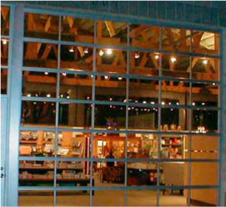
MULLION COLOR + STOREFRONT SYSTEM Natural annodized aluminum mullions. Clear glazing.
