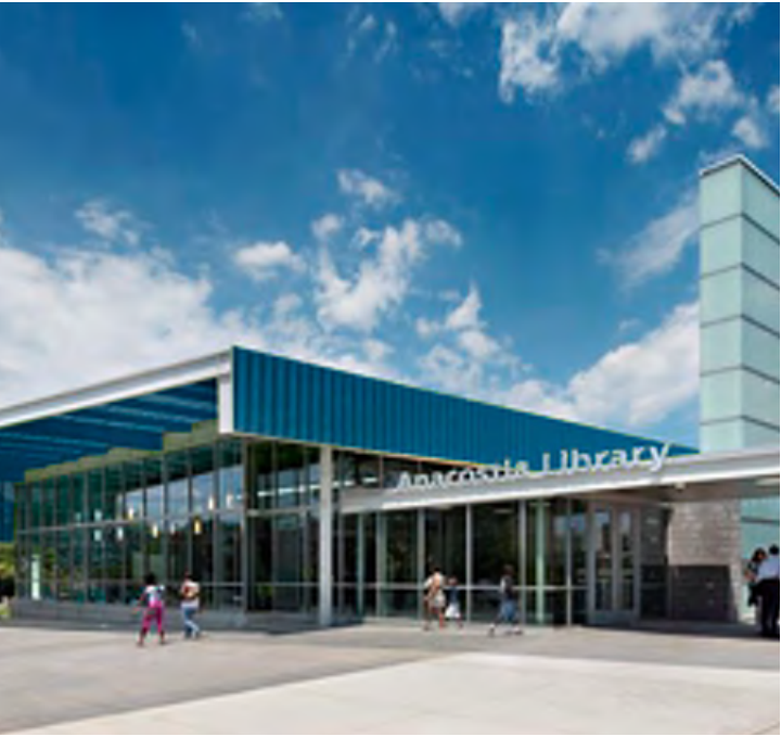
EYEBROW - DARK BLUE Morin: metal panels. Dark blue custom color, PMS 2188 part solid / part perforated.
