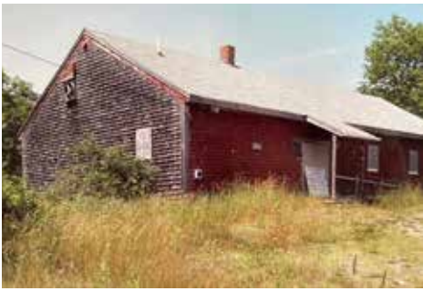
A mill building built in 1912 which used to sit on the Dennys River, but got moved across the street in 1930.
