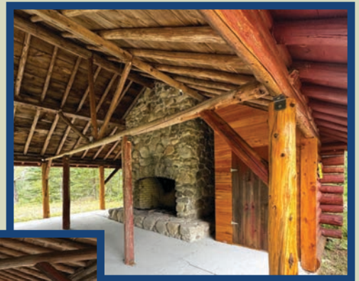
The DSF's Dennys River Sportsman's Club was rehabilitated in 2024 and is now a picnic pavilion with a concrete floor and a stone masonry hearth fireplace and metal roof.
