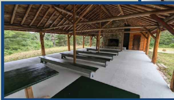
The DSF's Dennys River Sportsman's Club was rehabilitated in 2024 and is now a picnic pavilion with a concrete floor and a stone masonry hearth fireplace and metal roof.
