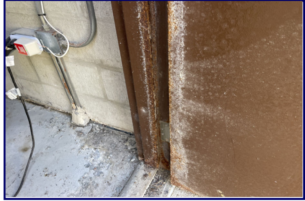
Photograph 5.8: Door jamb corrosion.
