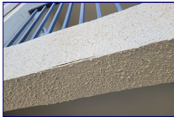
Photograph 5.12: Corridor beam spall.
