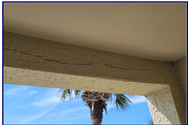
Photograph 5.16: Balcony beam spall.
