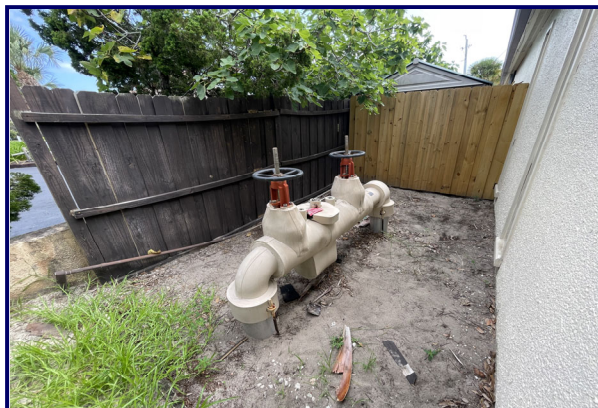
Photograph 5.11: Primary backflow preventer.
