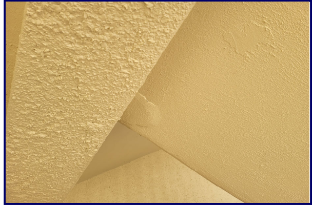
Photograph 5.14: Concrete stair spall.
