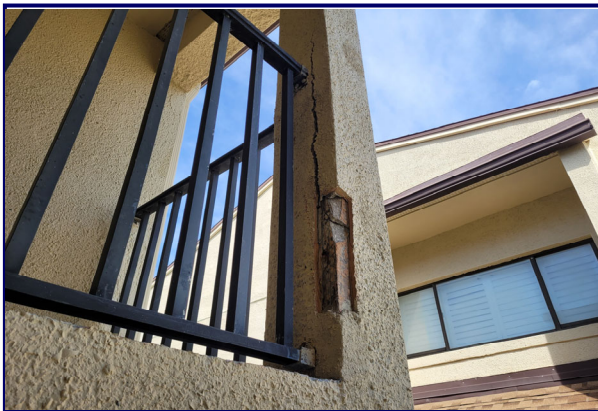
Photograph 5.15: Column spall.
