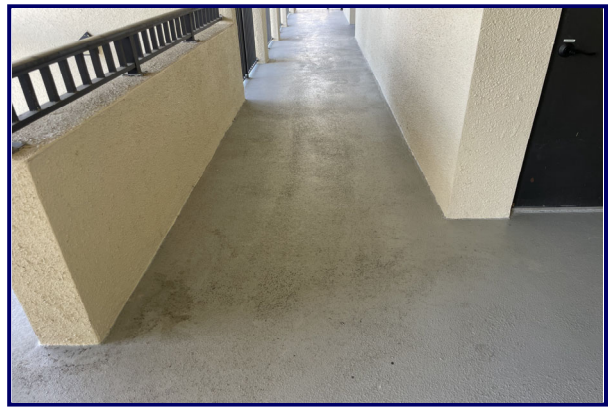
Photograph 5.10: Building corridor with polyurethane deck coating.
