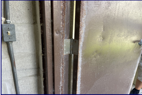
Photograph 5.7: Steel utility door with corrosion.
