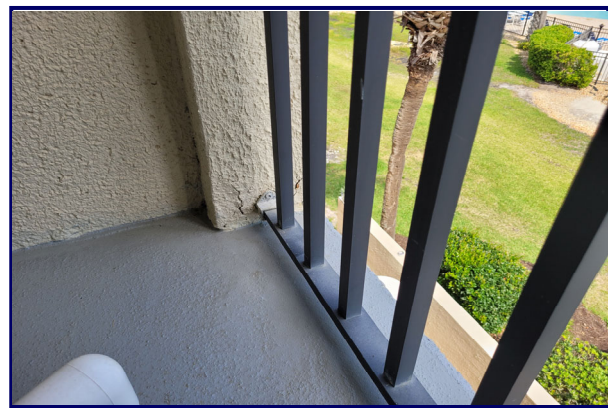
Photograph 5.18: Spall at rail base.
