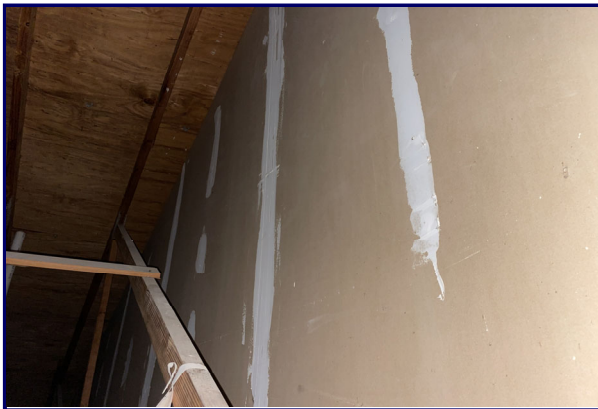
Photograph 5.9: Typical unit attic fire wall partition.
