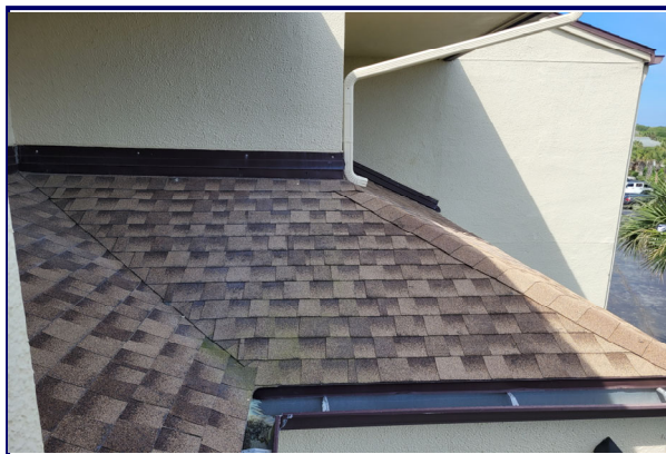
Photograph 5.17: Architectural shingle roofing.
