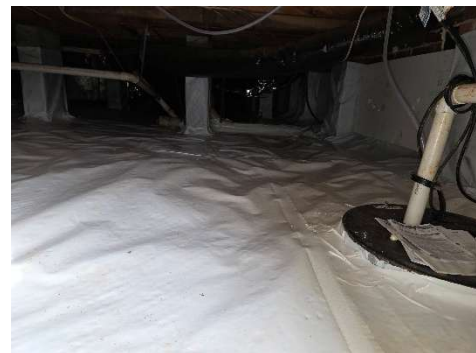
Newly Encapsulated Crawl Space
