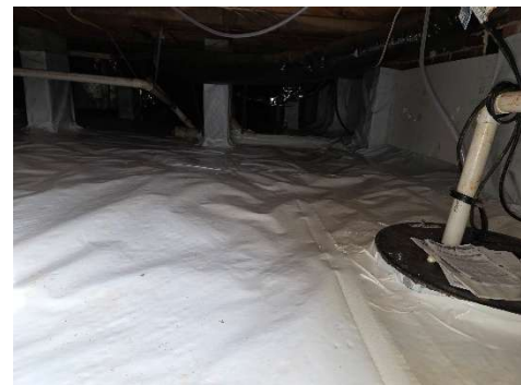
Newly Encapsulated Crawl Space
