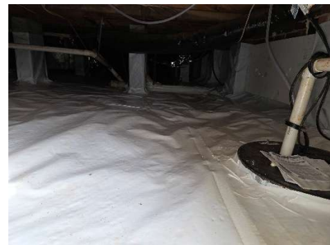
Newly Encapsulated Crawl Space
