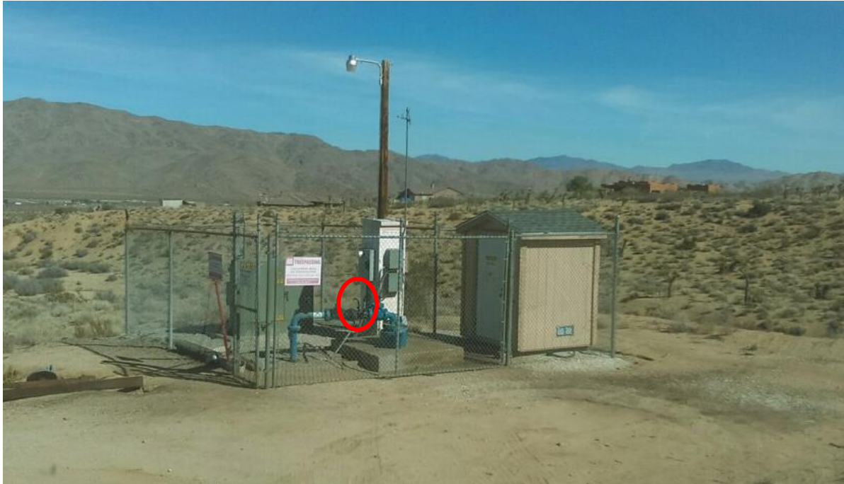
Figure 4: Example of a District Wellhead with Sampling Tap
