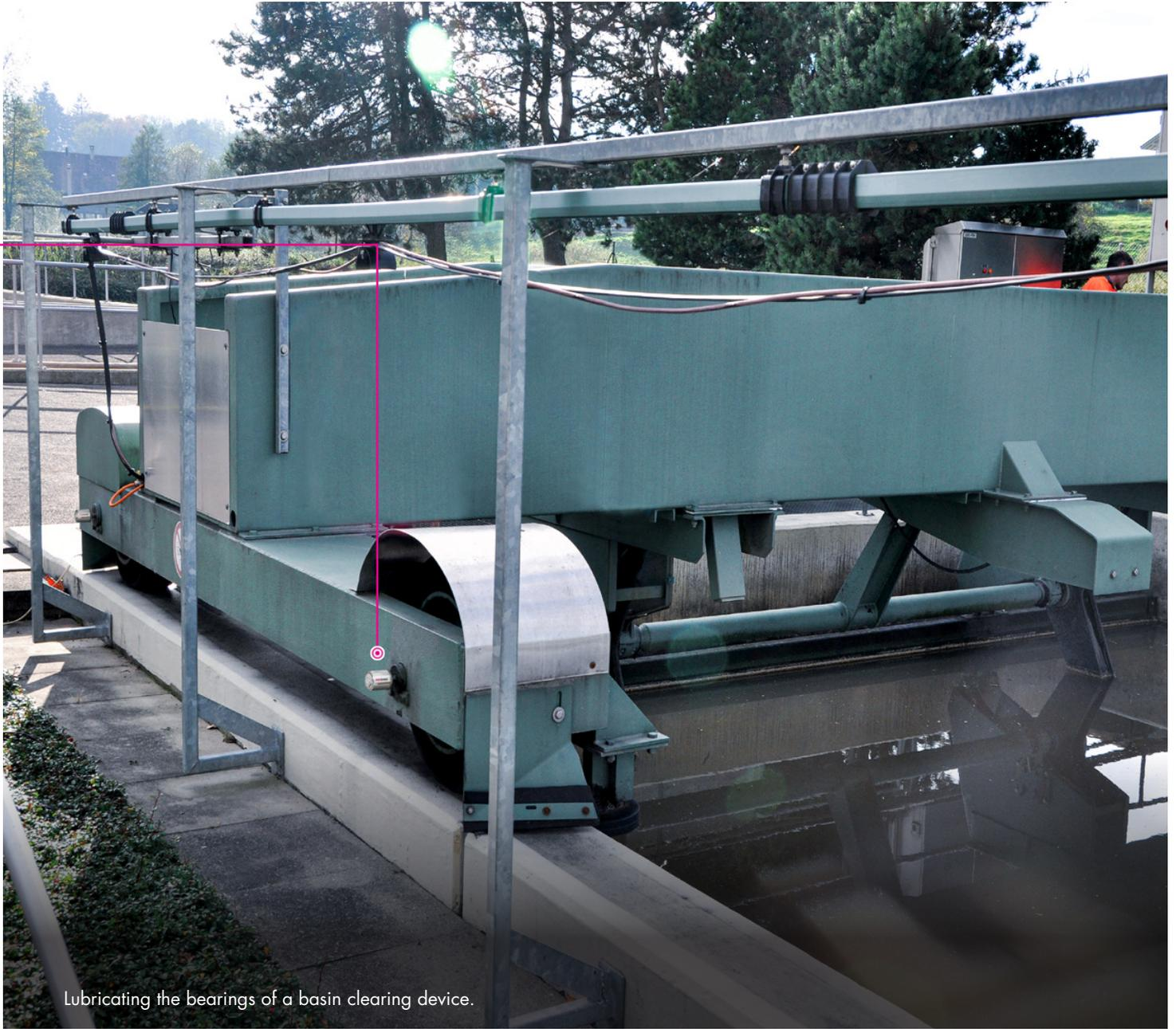
Lubricating the bearings of a basin clearing device.
