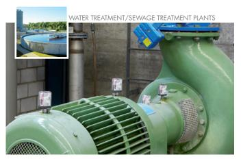
60 ml lubricators on the electric motor and the drive shaft ensure continuous lubrication of a centrifugal pump.
