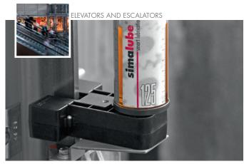
The 125 ml simalube maintains the guide rails of elevators and prevents dry friction. The system is attached directly to the cabin roof.
