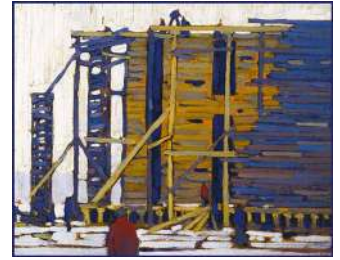
Building the Ice House, Hamilton, 1912 LH-020
