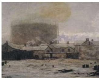
The Gas Works LH-110
