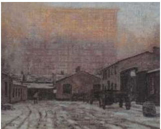
The Eaton Manufacturing Building, 1911 LH-109
