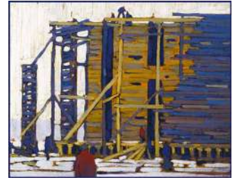
Building the Ice House, Hamilton, 1912 LH-020
