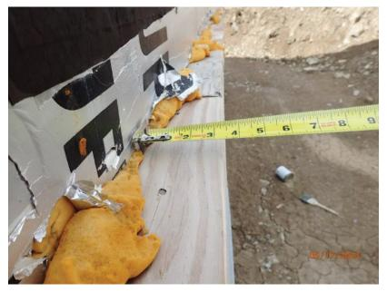
May 17, 2023, Disc OBS1, Photograph 54, DLC, 101 Mule Deer Court, modular units mis-aligned with the foundation wall at west half.
