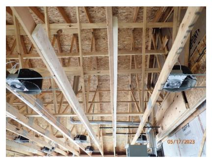
May 17, 2023, Disc OBS1, Photograph 103, DLC, 101 Mule Deer Court, repairs at bottom chord of garage trusses.
