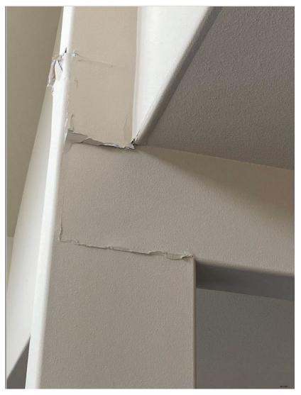
Interior damages related to the setting of the modular components and foundation movement or interior post issues (Bates Number Smith\_000521).
