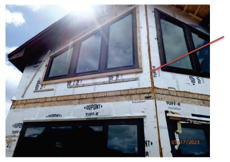
May 17, 2023, Disc OBS1, Photograph 49, DLC, 101 Mule Deer Court, east half of the north elevation showing incomplete modular unit installation and 2-inch gap at centerline.
