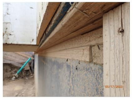
May 17, 2023, Disc OBS1, Photograph 72, DLC, 101 Mule Deer Court, overhang of modular unit to foundation wall east elevation.
