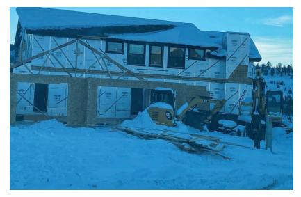
Owner provided photo, trusses and other building materials stored directly on the ground without dunnage with no protective covering, and covered with snow and ice.
