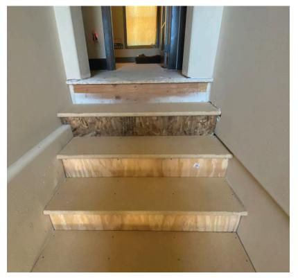
Owner provided photo prior to the re-framing showing non-compliant dimensional variance between the treads and risers at the second floor.
