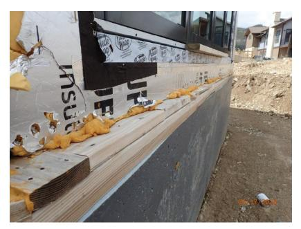
May 17, 2023, Disc OSB1, Photograph 53, DLC, 101 Mule Deer Court, modular units mis-aligned with the foundation wall.
