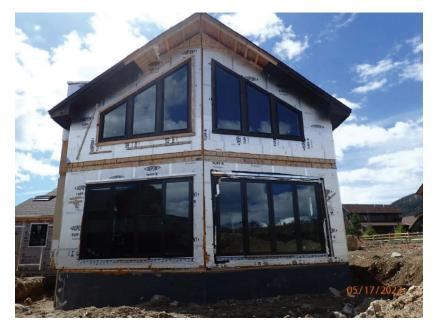
May 17, 2023, Disc OBS1, Photograph 11, DLC, 101 Mule Deer Court, overall view of the north elevation. 2x12 band board is missing at second story floor line.
