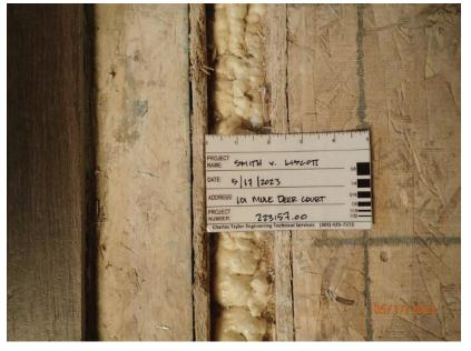
May 17, 2023, Disc OBS1, Photograph 242, DLC, 101 Mule Deer Court, 2-inch gap between units filled with spray foam at sill into upstairs Bath #4.
