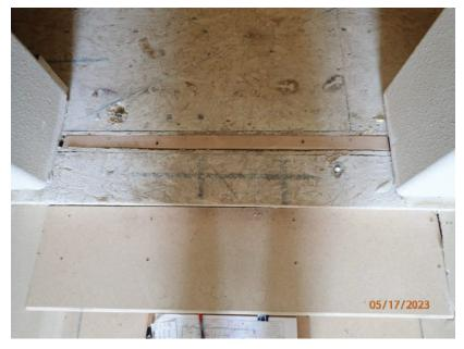
May 17, 2023, Disc OBS1, Photograph 227, DLC, 101 Mule Deer Court, 2-inch gap between east and west unit at subfloor at top of stairs.
