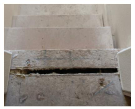
Owner provided photo showing the 2-inch gap at the mating line between the modular units. Top of stairs at second floor level.
