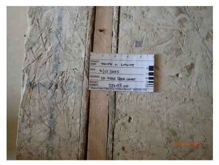
May 17, 2023, Disc OBS1, Photograph 228, DLC, 101 Mule Deer Court, 2x lumber used to fill to gap between the east and west modular units. The lumber does not sufficiently fill the gap.
