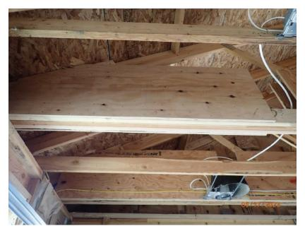
May 17, 2023, Disc OBS1, Photograph 106, DLC, 101 Mule Deer Court, repairs at bottom chord of garage trusses.
