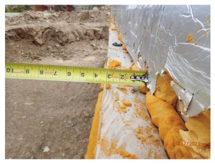
May 17, 2023, Disc OBS1, Photograph 65, DLC, 101 Mule Deer Court, modular units mis-aligned with the foundation wall at east half.
