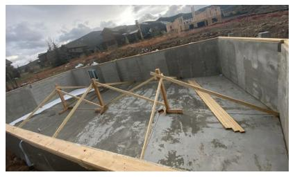
Owner provided photo showing the use of dimensional lumber supports for the structural steel beam. Note there is no lateral support provided for the basement walls that would be necessary to backfill them prior to the modulars being set.
