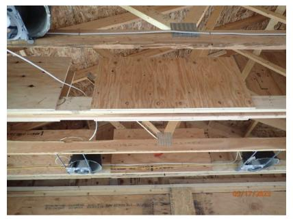
May 17, 2023, Disc OBS1, Photograph 107, DLC, 101 Mule Deer Court, repairs at bottom chord of garage trusses.
