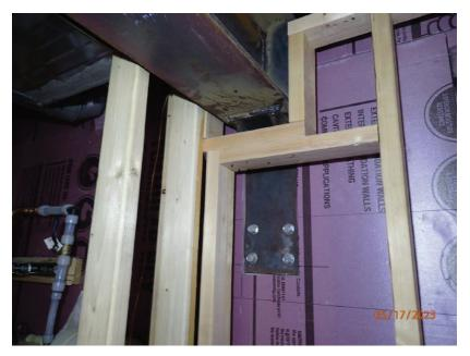
May 17, 2023, Disc OBS1, Photograph 126, DLC, 101 Mule Deer Court, approved beam bearing seat as installed at the south and north foundation wall bearing points.
