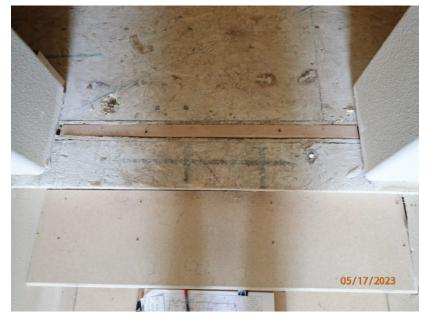
May 17, 2023, Disc OBS1, Photograph 227, DLC, 101 Mule Deer Court, 2-inch gap at top of stairs, 2x lumber used to fill to gap between the east and west modular units.
