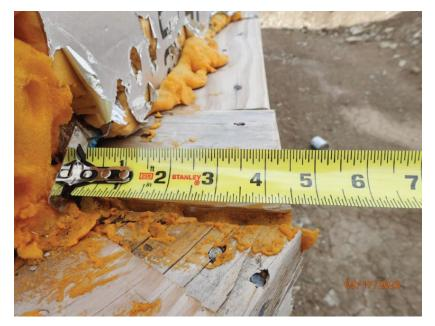
May 17, 2023, Disc OBS1, Photograph 55, DLC, 101 Mule Deer Court, modular units mis-aligned with the foundation wall at west half.
