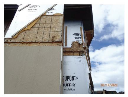
May 17, 2023, Disc OBS1, Photograph 69, DLC, 101 Mule Deer Court, damage at NE corner from use of a mini-excavator pushing on the units.
