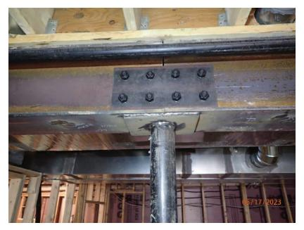
May 17, 2023, Disc OBS1, Photograph 125, DLC, 101 Mule Deer Court, approved beam splice plate installed at the south beam support location.
