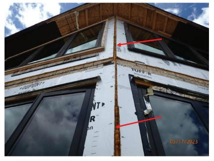
May 17, 2023, Disc OSB1, Photograph 52, DLC, 101 Mule Deer Court, gap between east and west modular units. Gap offset between upper and lower levels.
