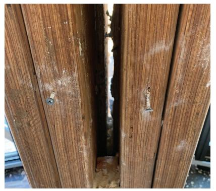
Owner provided photo showing the gap between the modular units prior to Liscott's application of spray foam insulation in this gap.
