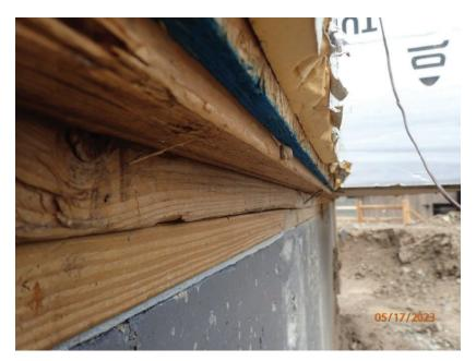
May 17, 2023, Disc OBS1, Photograph 73, DLC, 101 Mule Deer Court, overhang of modular unit to foundation wall east elevation.
