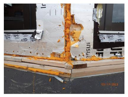
May 17, 2023, Disc OSB1, Photograph 51, DLC, 101 Mule Deer Court, 2-inch gap between east and west modular units gap filled with spray foam.
