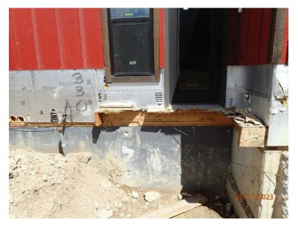
May 17, 2023, Disc OBS1, Photograph 21, DLC, 101 Mule Deer Court, south elevation entry foundation and porch framing have been removed.
