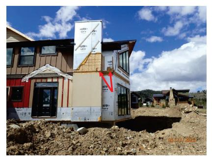
May 17, 2023, Disc OBS1, Photograph 12, DLC, 101 Mule Deer Court, modular unit construction and damage at NE corner from use of a mini-excavator.
