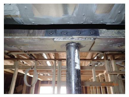
May 17, 2023, Disc OBS1, Photograph 124, DLC, 101 Mule Deer Court, repaired connection between support post and steel beam. This attachment detail was done at both the north and south support post. North post location does not have a splice connection plate.
