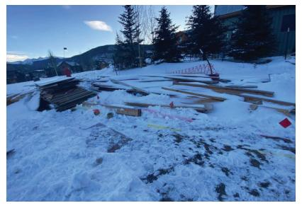
Owner provided photo, trusses and other building materials stored directly on the ground without dunnage with no protective covering, and covered with snow and ice.
