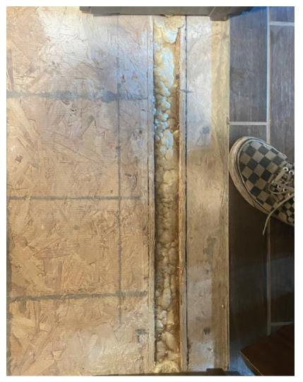
Owner provided photo showing spray foam insulation applied in the 2-inch gap at the mating line between the modular units at the first floor.
