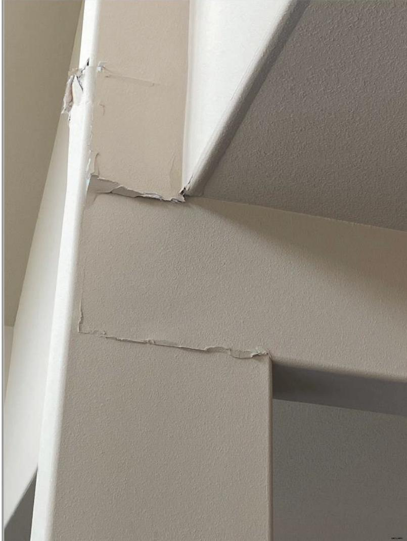
Interior damages related to the setting of the modular components and foundation movement or interior post issues (Bates Number Smith\_000521).
