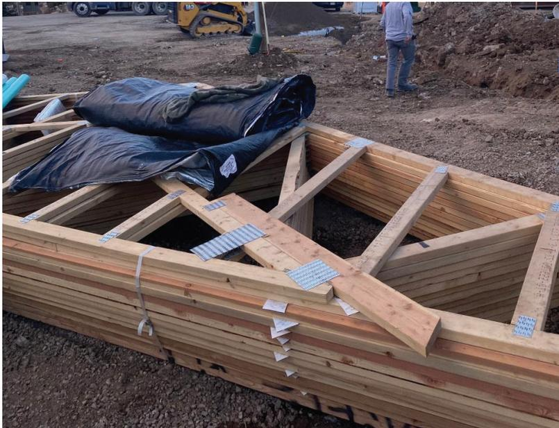
Owner provided photo, trusses delivered to the site and stored directly on the ground without dunnage.
