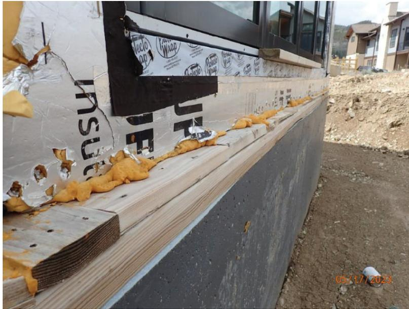
May 17, 2023, Disc OSB1, Photograph 53, DLC, 101 Mule Deer Court, modular units mis-aligned with the foundation wall.
