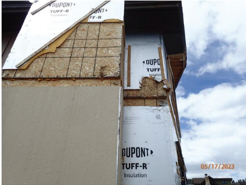
May 17, 2023, Disc OBS1, Photograph 69, DLC, 101 Mule Deer Court, damage at NE corner from use of a mini-excavator pushing on the units.
