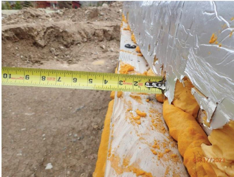
May 17, 2023, Disc OBS1, Photograph 65, DLC, 101 Mule Deer Court, modular units mis-aligned with the foundation wall at east half.
