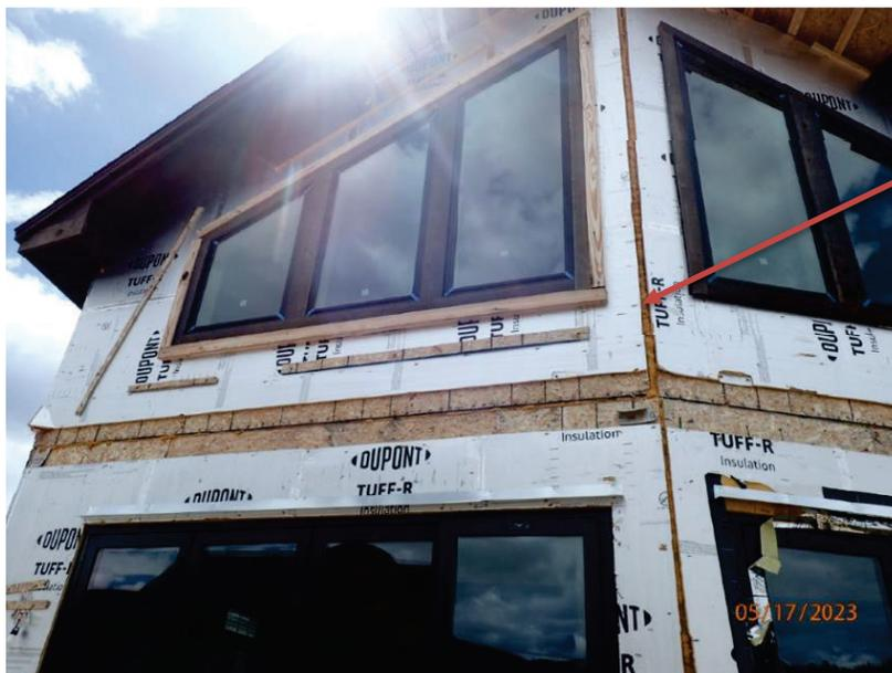
May 17, 2023, Disc OBS1, Photograph 49, DLC, 101 Mule Deer Court, east half of the north elevation showing incomplete modular unit installation and 2-inch gap at centerline.
