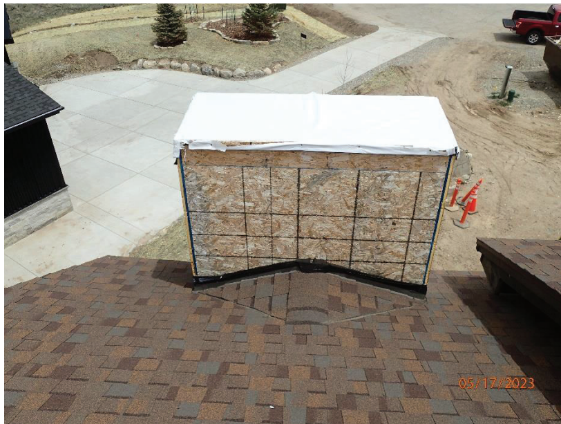
May 17, 2023, Disc OBS1, Photograph 291, DLC, 101 Mule Deer Court, missing weather protection, WRB, trim and siding.
