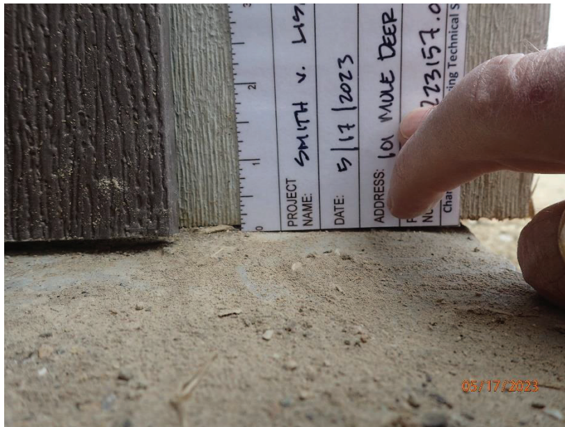
May 17, 2023, Disc OBS1, Photograph 88, DLC, 101 Mule Deer Court, trim tight to concrete at garage door jamb.
