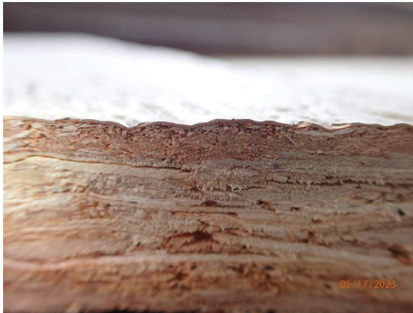
May 17, 2023, Disc OBS1, Photograph 276, DLC, 101 Mule Deer Court, untreated cut ends of vertical batten.
