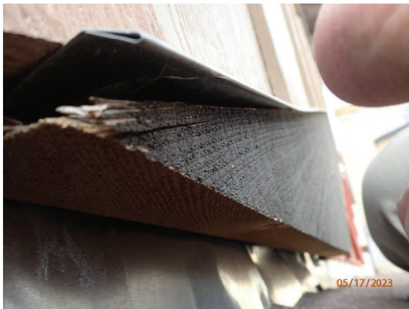
May 17, 2023, Disc OBS1, Photograph 274, DLC, 101 Mule Deer Court, untreated cut ends and cut siding edges.
