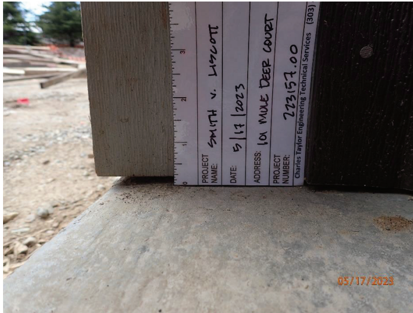
May 17, 2023, Disc OBS1, Photograph 87, DLC, 101 Mule Deer Court, trim tight to concrete at garage door jamb.
