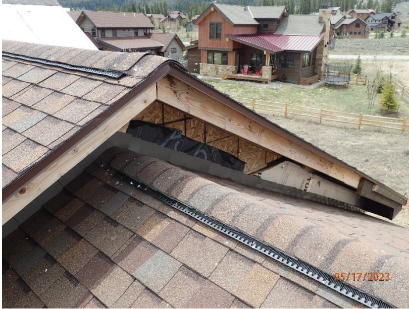
May 17, 2023, Disc OBS1, Photograph 292, DLC, 101 Mule Deer Court, missing trim and siding.
