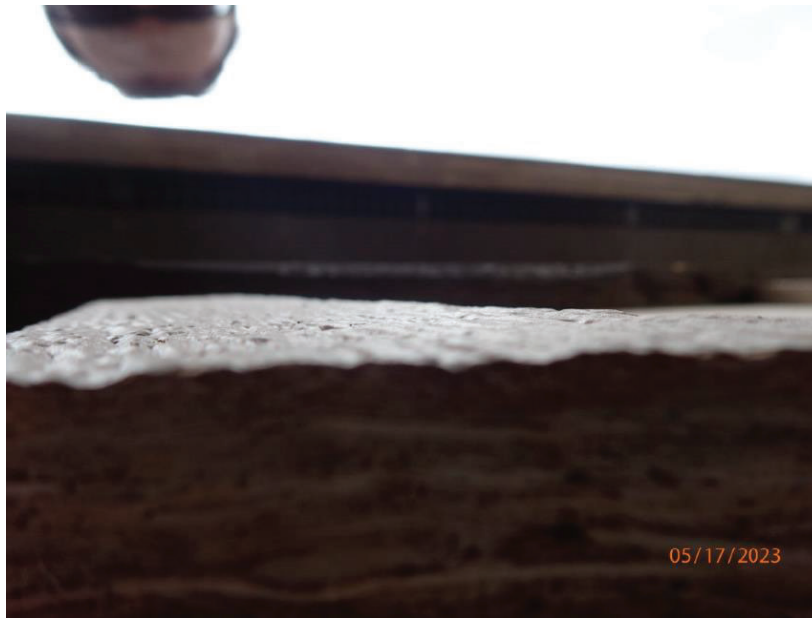
May 17, 2023, Disc OBS1, Photograph 275, DLC, 101 Mule Deer Court, untreated cut ends of vertical batten.
