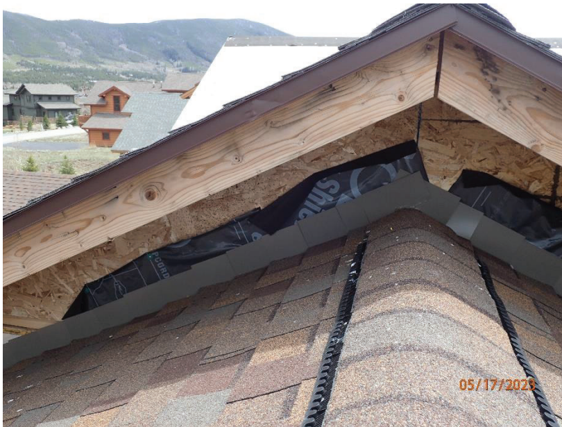
May 17, 2023, Disc OBS1, Photograph 293, DLC, 101 Mule Deer Court, missing trim and siding.
