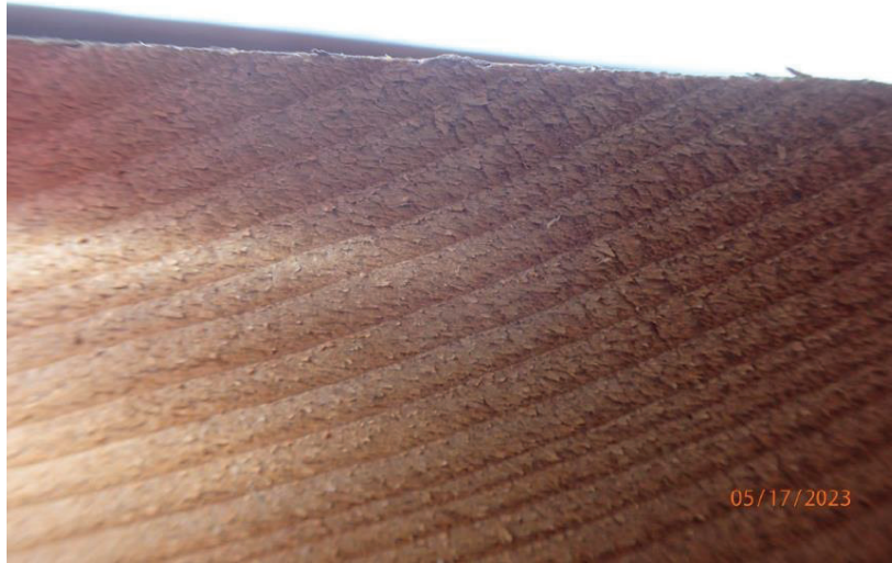
May 17, 2023, Disc OBS1, Photograph 277, DLC, 101 Mule Deer Court, untreated cut ends of vertical batten.
