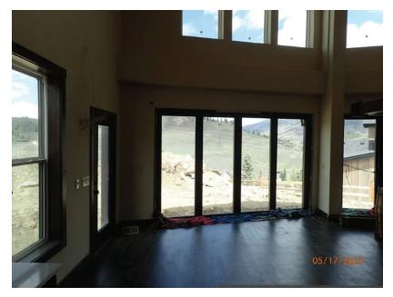
May 17, 2023, Disc OBS1, Photograph 157, DLC, 101 Mule Deer Court, unprotected finish flooring in the living/dining room area. The surface has an uneven appearance due to being in an uncontrolled environment.
