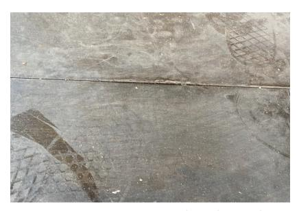
Owner provided photo showing damage to the finished flooring surface due to Liscott's failure to maintain proper protection during construction.
