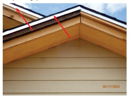
May 17, 2023, Disc OBS1, Photograph 85, DLC, p101 Mule Deer Court, incorrect drip edge metal installed. Design call for a pre-finished material.
