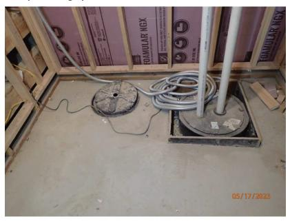
May 17, 2023, Disc OBS1, Photograph 135, DLC, 101 Mule Deer Court, radon system location in the basement. Owners paid to have the vent piping tied in at the basement ceiling.
