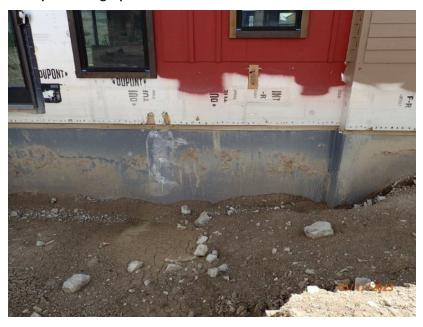
May 17, 2023, Disc OBS1, Photograph 37, 101 Mule Deer Court, the incorrect waterproofing materials applied to the foundation walls.
