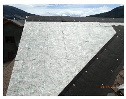
May 17, 2023, Disc OBS1, Photograph 289, DLC, 101 Mule Deer Court, exposed OSB at upper roof dormer. OSB is starting to swell and delaminate.
