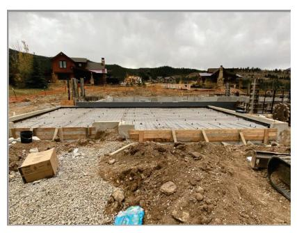
Garage floor formed and reinforcing placed without any drains or associated piping installed (Bates Number Smith\_000438).
