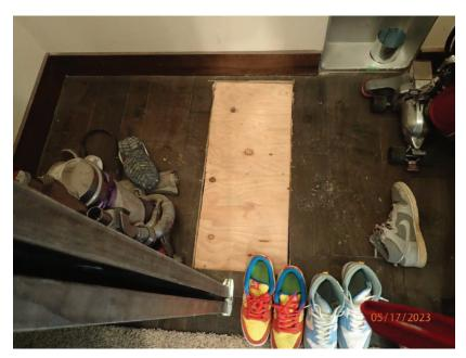
May 17, 2023, Disc OBS1, Photograph 216, DLC, 101 Mule Deer Court, area where flooring was removed as hole cut in the floor to access the water lines.
