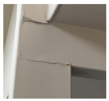
Owner provided photo showing damage to the drywall at the column in the Living/Dining area.
