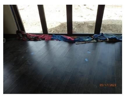
May 17, 2023, Disc OBS1, Photograph 172, DLC, 101 Mule Deer Court, unprotected finish flooring in the living/ dining room area. The blue tape marks locations of damage. The damage is related to the misaligned, and non-level foundation used to set the modular units.
