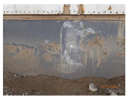
May 17, 2023, Disc OBS1, Photograph 38, 101 Mule Deer Court, the incorrect waterproofing materials were applied to the foundation walls.
