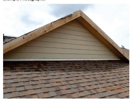
May 17, 2023, Disc OBS1, Photograph 284, DLC, 101 Mule Deer Court, incomplete roofing at dormers. Missing drip edge metal.
