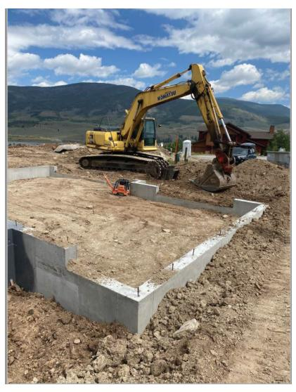
The garage was finished without any drain system.
