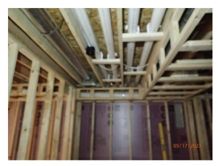
May 17, 2023, Disc OBS1, Photograph 139, DLC, 101 Mule Deer Court, rerouted furnace vent piping directed to the west elevation.
