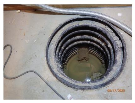
May 17, 2023, Disc OBS1, Photograph 136, DLC, 101 Mule Deer Court, sump pit location in the basement mechanical room. Pump has not been installed.
