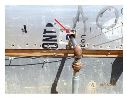
May 17, 2023, Disc OBS1, Photograph 24, DLC, 101 Mule Deer Court, gas line entry at south elevation of the residence. Line is being pulled down by pressure from the poorly compacted backfill material.
