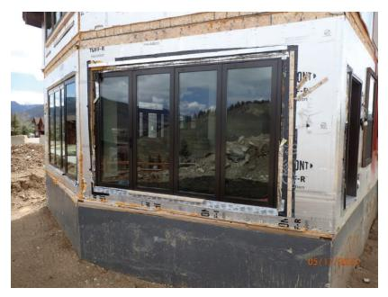
May 17, 2023, Disc OBS1, Photograph 46, 101 Mule Deer Court, the incorrect waterproofing materials were applied to the north elevation foundation walls.
