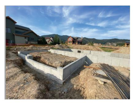
Owner provided photograph showing no coordinated drain or drywell was placed prior to the casting of the garage foundation.
