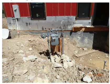
May 17, 2023, Disc OBS1, Photograph 23, DLC, 101 Mule Deer Court, gas meter at south elevation of the residence in poorly placed backfill zone.
