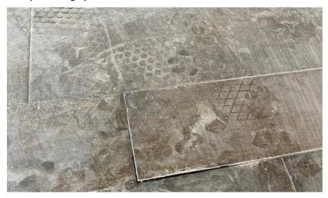
Owner provided photo showing damage to the finished flooring surface due to Liscott's failure to maintain proper protection during construction.
