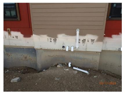
May 17, 2023, Disc OBS1, Photograph 36, DLC, 101 Mule Deer Court, rerouted furnace vent piping at the west elevation.
