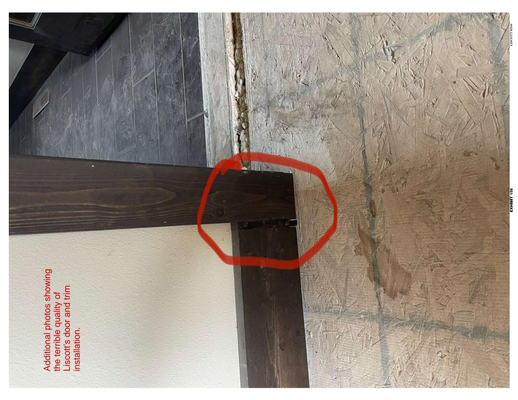
This image demonstrates, not only the terrible door and trim work performed by Liscott, but also how far out of plumb the walls are. Notice the shape and size of the scabbed in trim that had to be used to get the door to hang plumb
