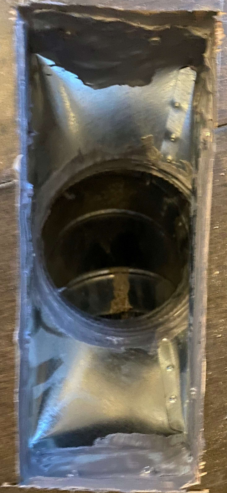
More examples of Liscotts ductwork installation
