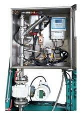
nents of the **Safety**Master system are mounted in a lockable cabinet which is protected against manipulation and installed on the separator unit.
