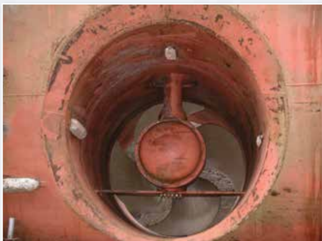
Example of corrosion in and around thruster tunnel.
