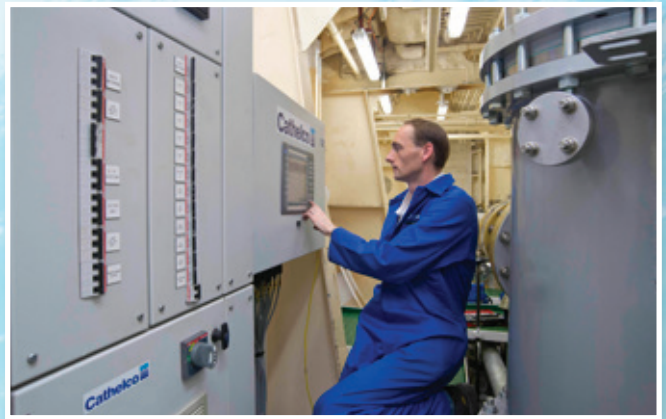
Automation control unit
