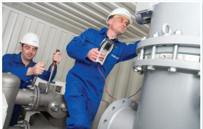
Work progresses on containerised system.
