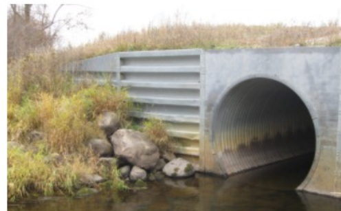
Retaining Wall and Erosion Control
