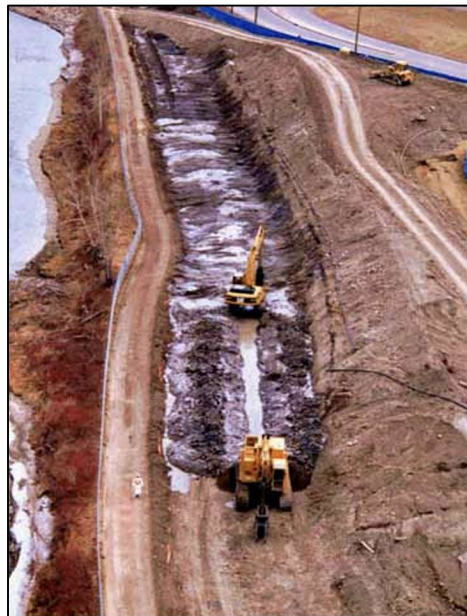
Figure 5.4: Construction of the containment cutoff wall.
