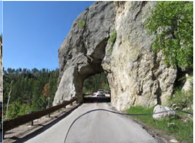
One of the one-lane tunnels
