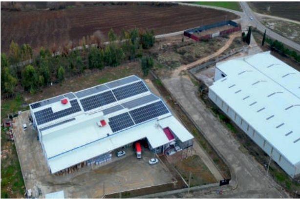
Multisistem SPP/ 850kWp
