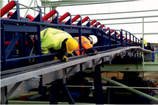
Cable Pulling Process
