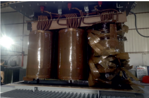
On-site Transformer Controls and Burnt Transformer Repair
